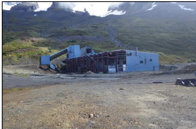
Figure 19.–Old mill building.
