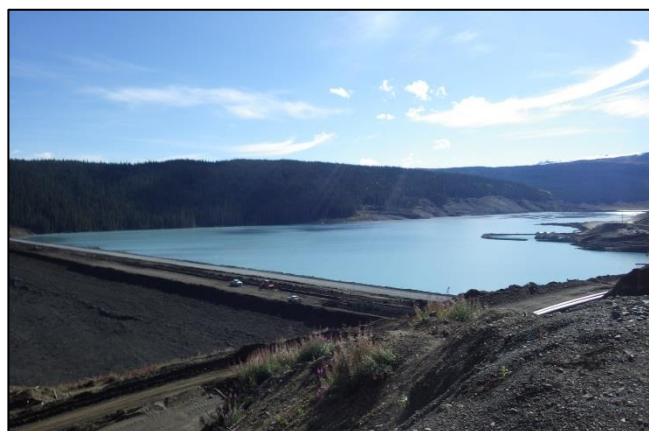
Figure 32.—Overview of the tailings impoundment area (North tailings dam in foreground).
