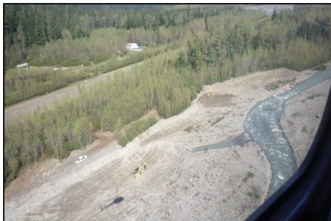
Figure 25.—Machinery stabilizing the bank of Bronson Creek.
