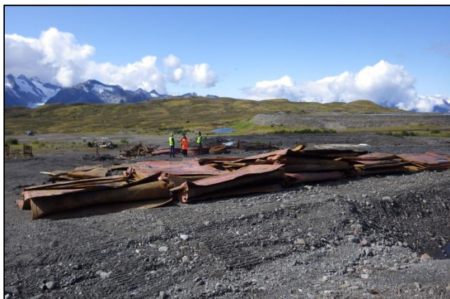
Figure 22.–Broken down tanks from tank farm staged for removal.
