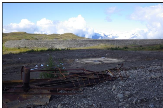
Figure 21.–Tank farm after tank removal.
