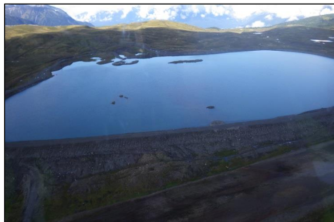
Figure 23.–Tailings storage facility.
